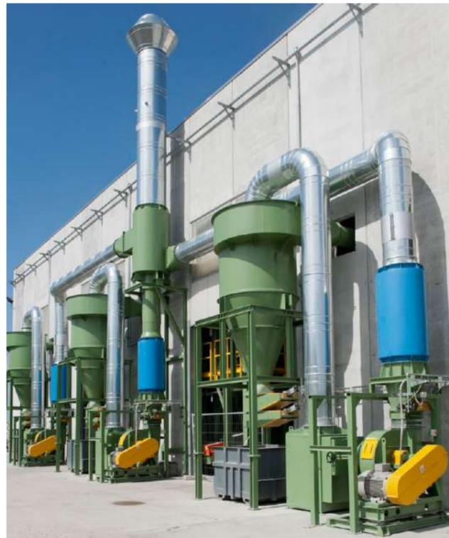
The cyclones are used as de-dusting dust collectors in industrial processes, where rough dust particles, chips, saw dust and other types of powders are treated.
